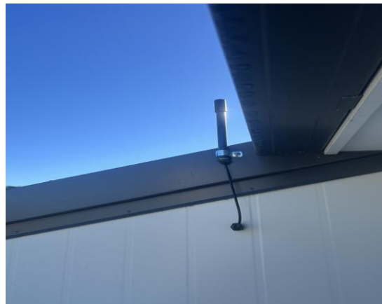
Antenna external installation
